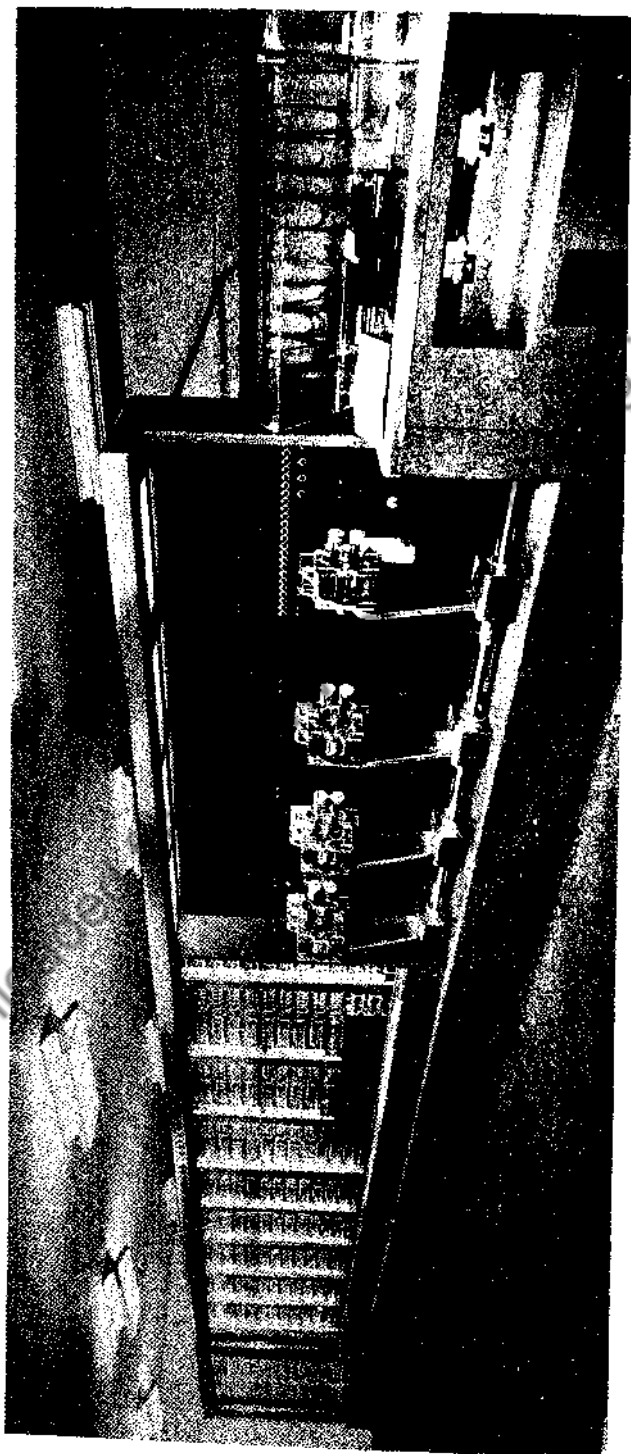
FIG. 45. General front view of automatic sequence-controlled calculator (Harvard Mark I Calculator).
